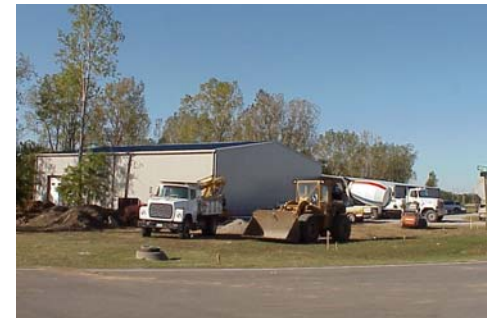
Control Vision Corp. - Pittsburg, New building expansion in North Industrial Park
