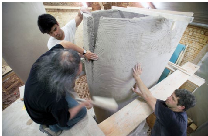
Top: Jun on Scaffolding. 2006–2007. With studio assistant building Dangos. Pittsburg, Kansas.
